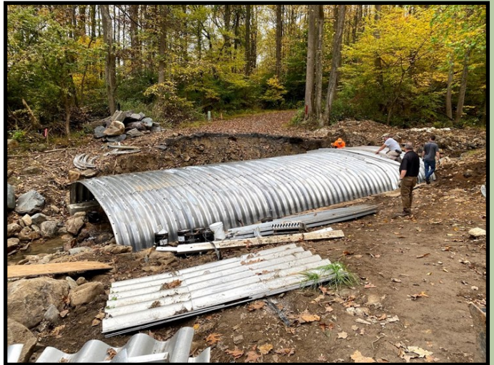
At right: Durham Township and representatives from Lane Enterprises, Inc. building the metal bottomless arch pipe in the open streambed
