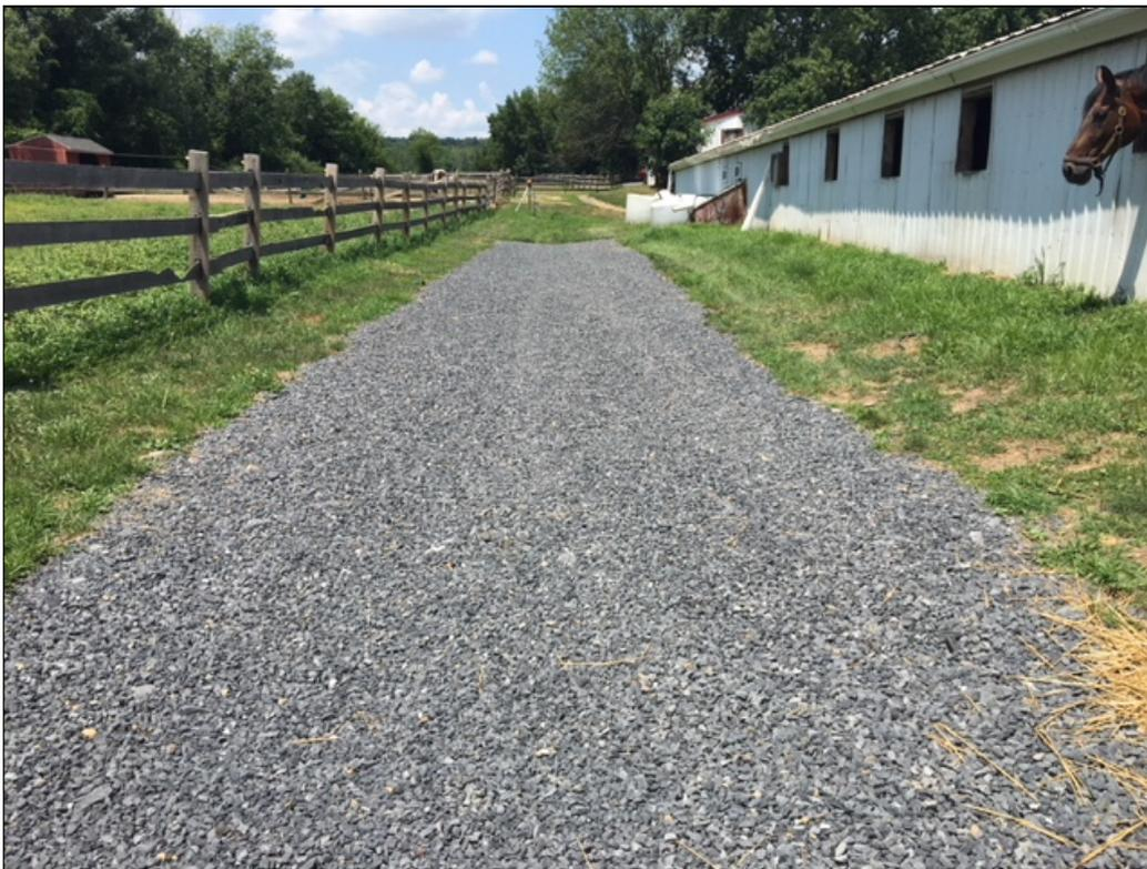
Photo 12. Waterway #2 after repair to rock-lined and looking up to Waterway #1 (WIP Participant #5).
