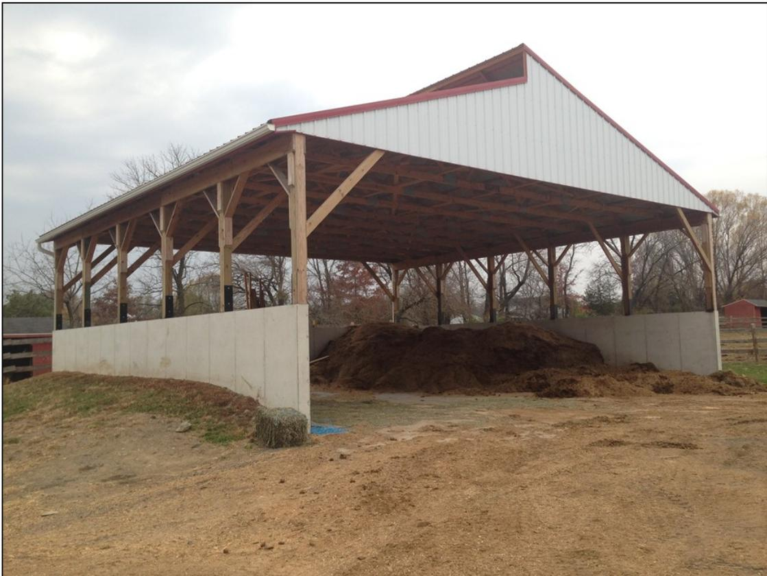
Photo 8. Roofed stack pad shortly after construction (WIP Participant #5).
