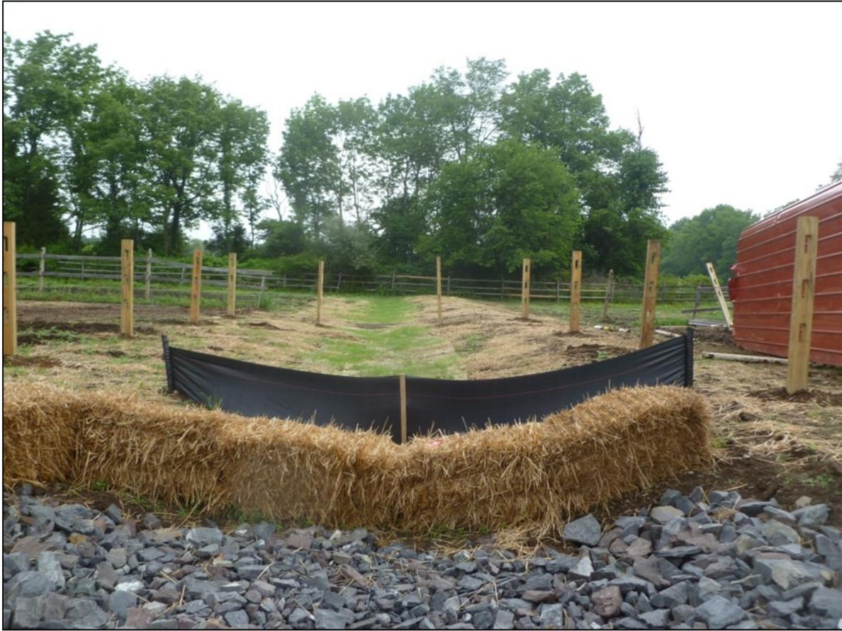
Photo 9. Grassed diversion #3 and rock outlet stabilization (WIP Participant #5).
