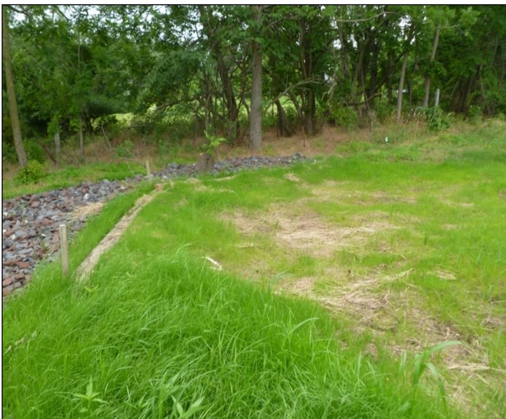
Photo 6. Infiltration bed and level lip spreader shortly after construction (WIP Participant #44).
