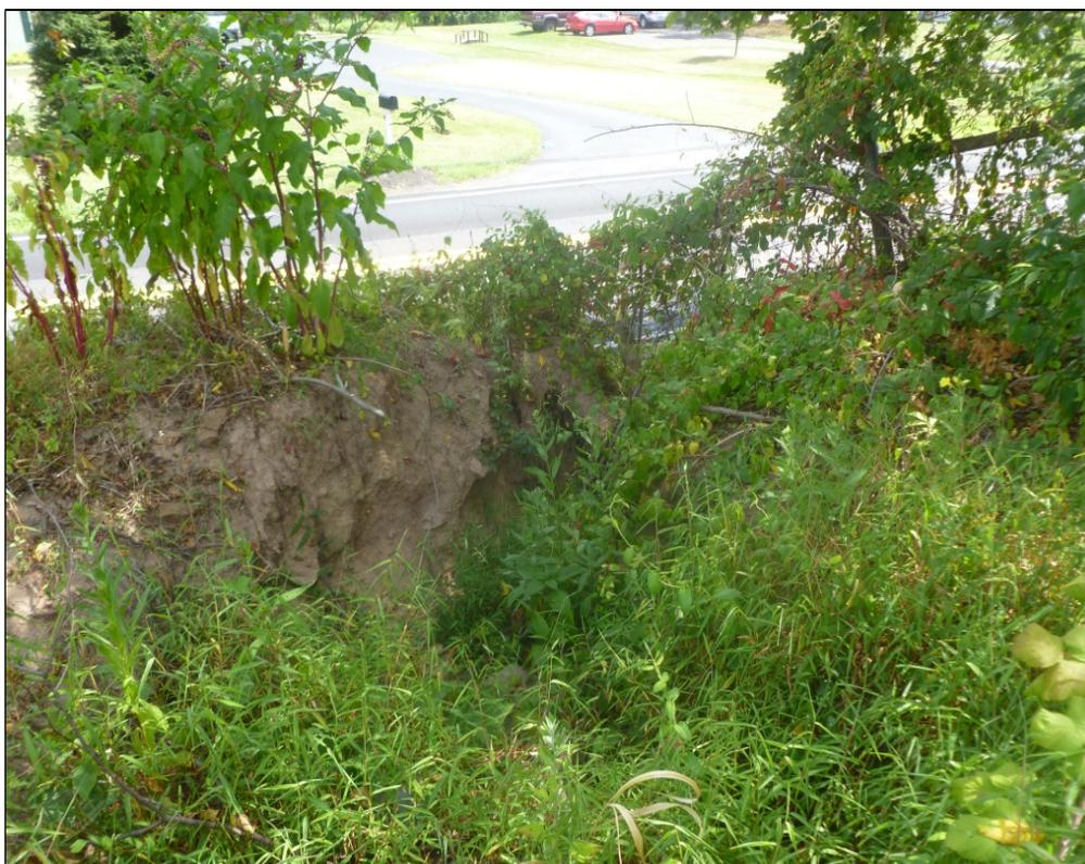
Photo 5. Erosion on Ferry Rd embankment before infiltration bed and level lip spreader install (WIP Participant #44).
