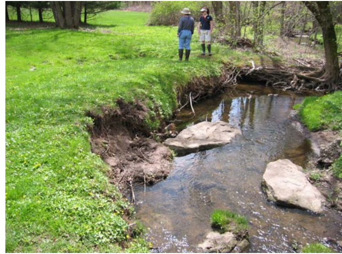
NPS 5 (Below Bridge)
