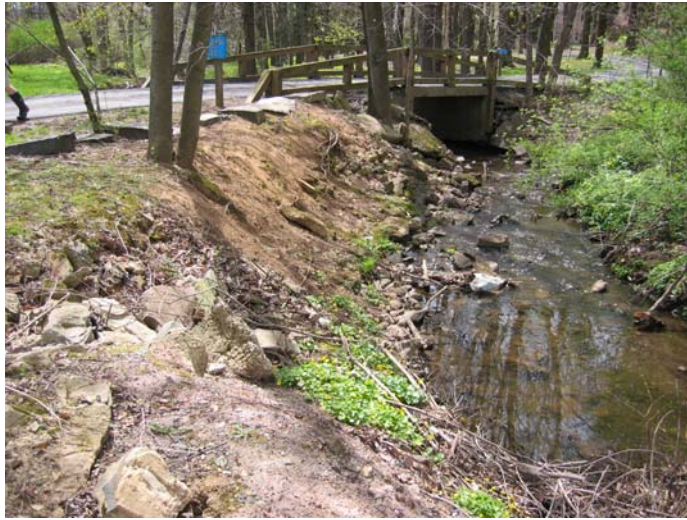
NPS 5 (Above Bridge)
