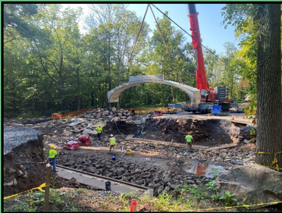
Above: one section of the Rosenberger Road bridge being set by crane during construction 2021.
