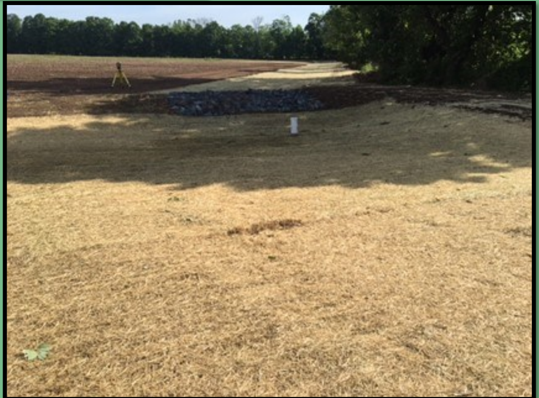
Photo to the right: a Water & Sediment Control basin and downslope grass waterway. This was installed to eliminate accelerated soil erosion that was occurring in the crop field.
