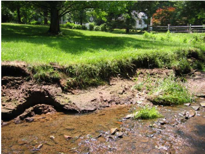
NPS Problem 15 (Second View)
