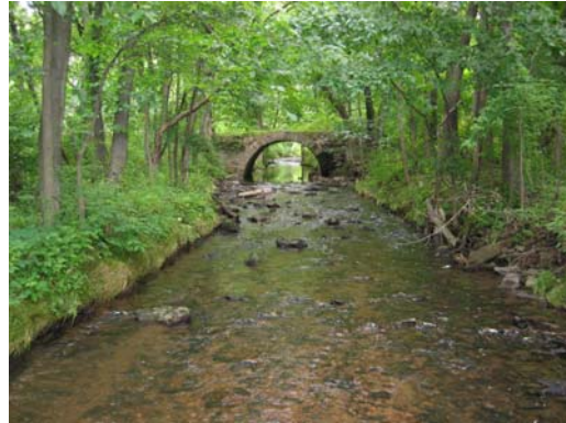
Scenic Section of Cooks Run in the Lower Subwatershed Area
