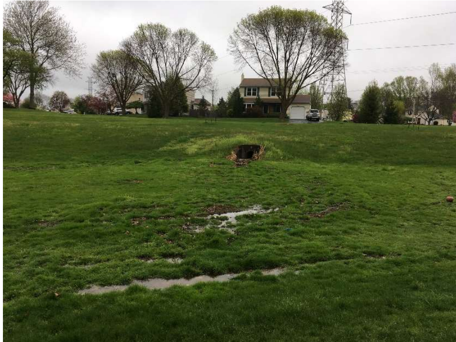
Figure 2.4.24 – 2.4.25: Site conditions at Adeline Place and Barnsbury Road stormwater basin.
