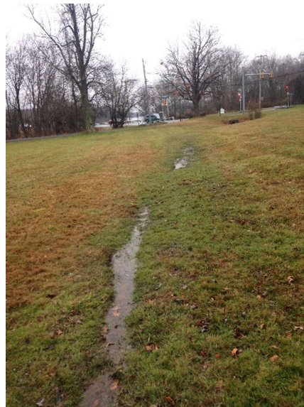
Figure 2.4.1: Channel condition at Ellis Road.
