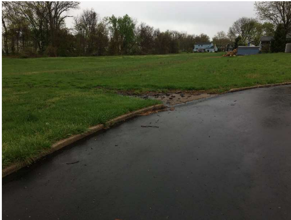
Figure 2.4.26: Site conditions at Argyle Road stormwater basin.
