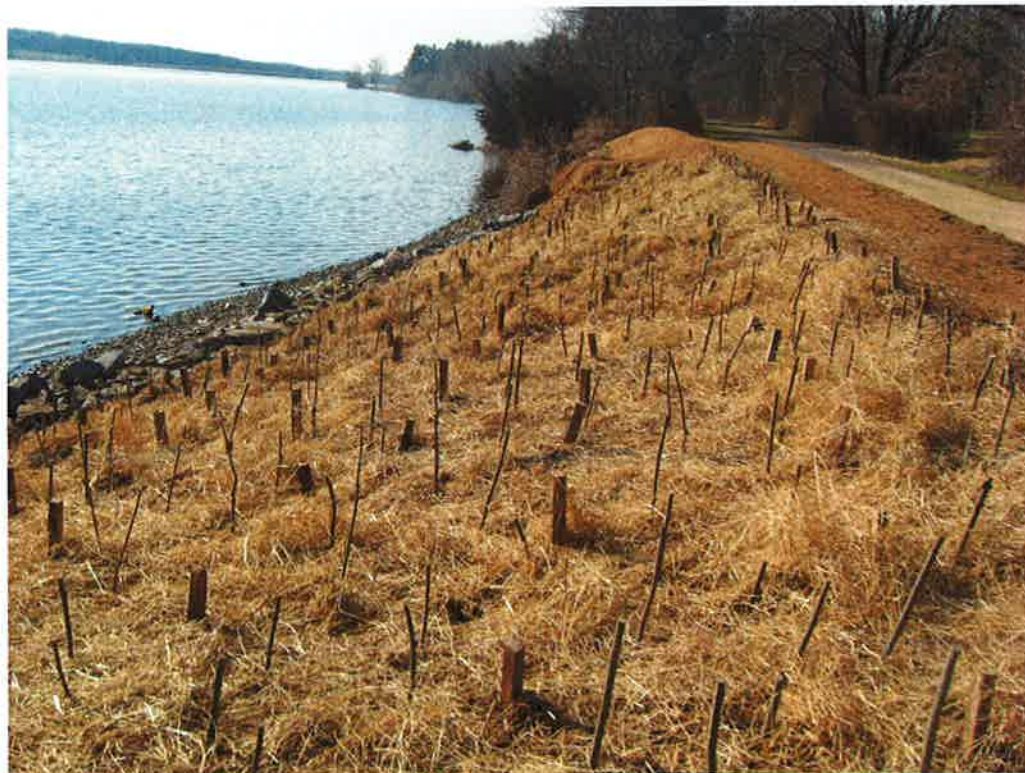
Photo 6. Newly restored bank after final stabilization
