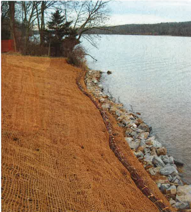
Photo 4. Installation of coir matting and live fascines.
