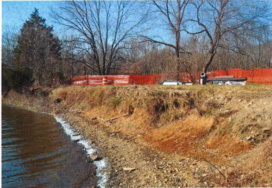
Photo 1. Project area immediately before start of construction
