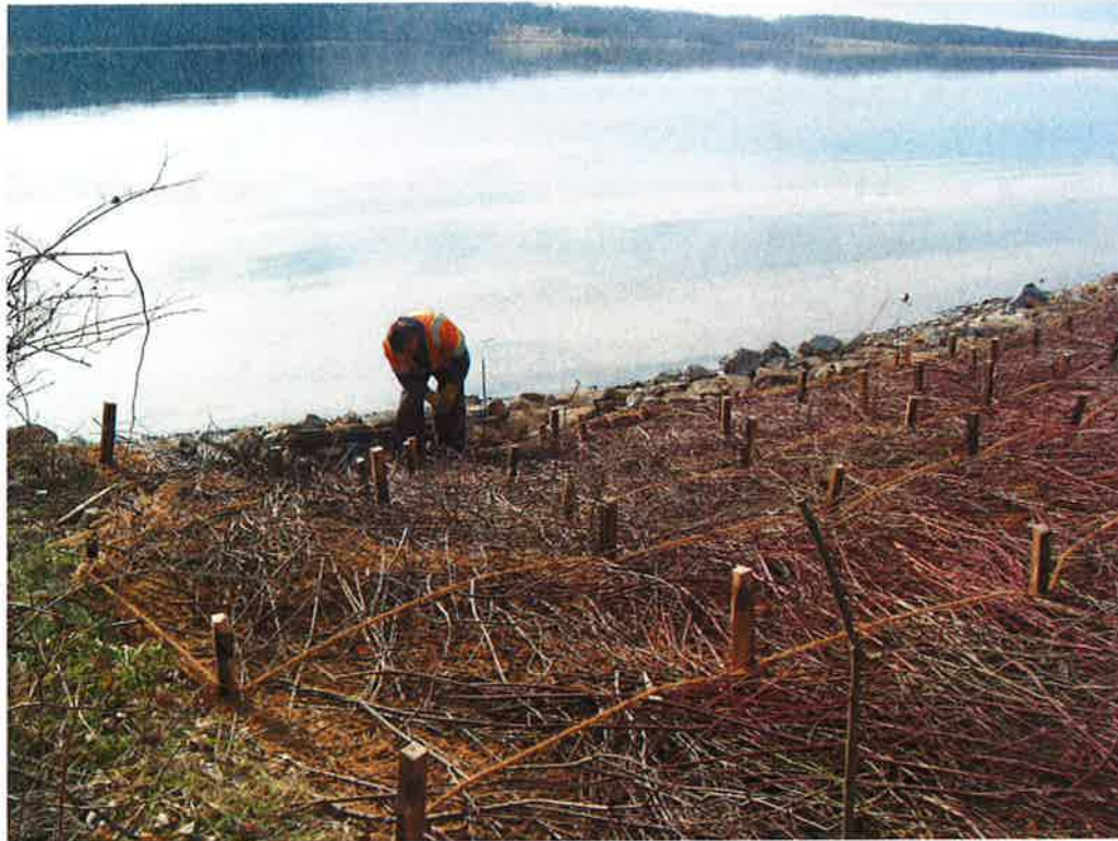
Photo 5. The crew secures the brush mattresses and installs live stakes
