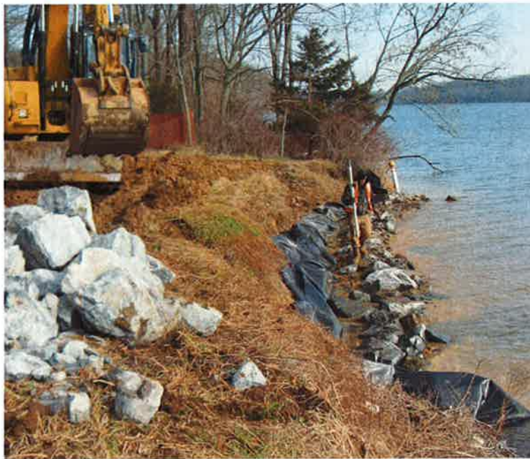
Photo 2. Placement of geotextile and boulder toe protection.
