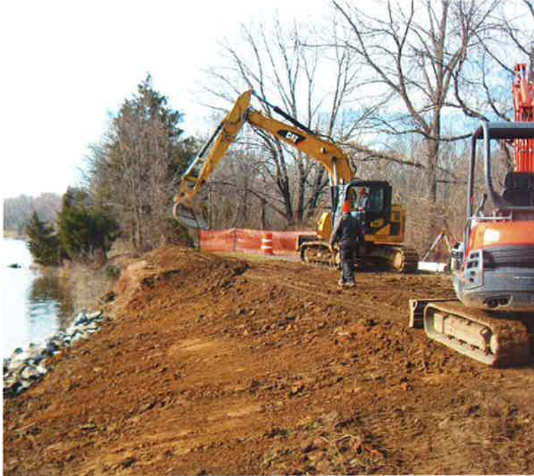
Photo 3. Enviroscapes, Inc. crew regrading bank
