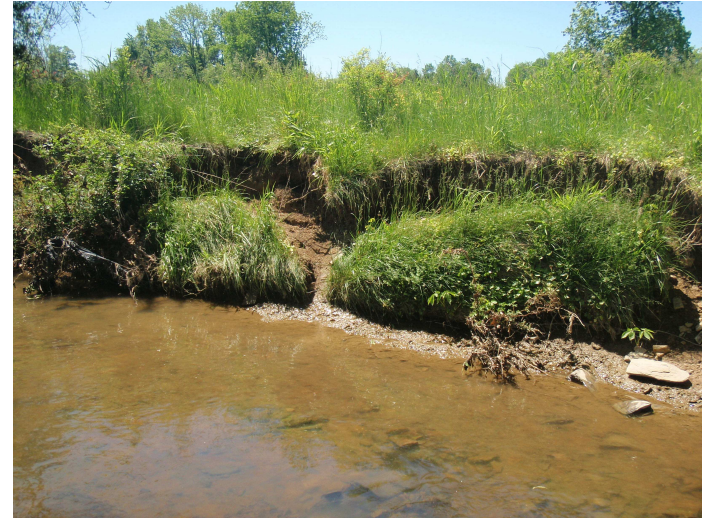
Problem Area – PD2
