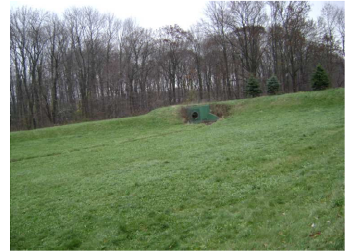
No.28 - Photograph 1 Estates at Brookside – Basin 2
