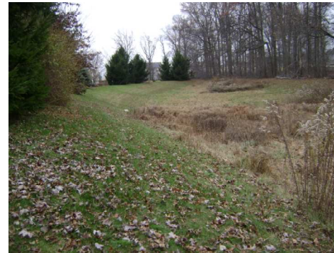
No.30 - Photograph 1 Country Greene Subdivision – Basin 1
