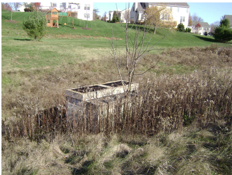
No.16 - Photograph 1 Windtree Subdivision – Water Quality Basin 3
