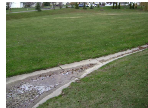
No.31 - Photograph 1 Country Greene Subdivision – Basin 2
