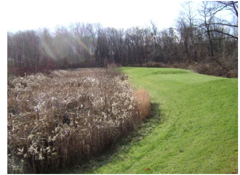
No.34 - Photograph 1 Central Bucks Elementary School along Route 611
