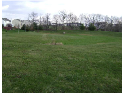
No.14 - Photograph 1 Windtree Subdivision – Water Quality Basin 1
