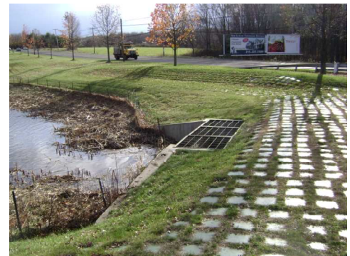
No.18 - Photograph 1 Bucks Country Gardens – Regional Wet Pond
