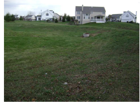
No.15 - Photograph 1 Windtree Subdivision – Water Quality Basin 2
