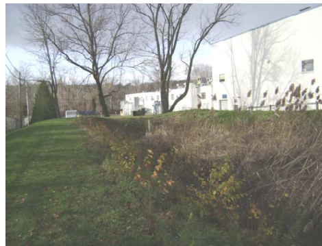
No.36 - Photograph 1 Penn Engineering – Basin 2
