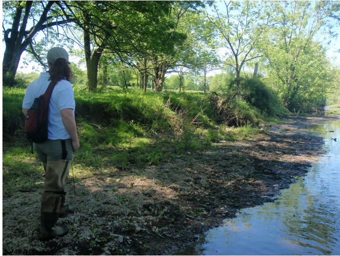
Problem Area – PD1
