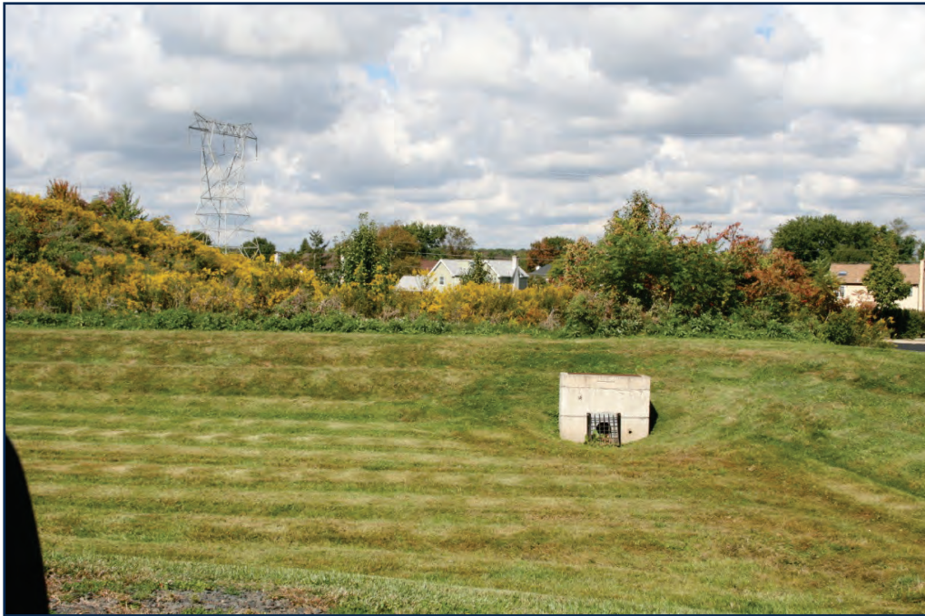
Figure 13: Detention basin that could be retrofitted along Route 263 (Fish Creek) (September 2013)
