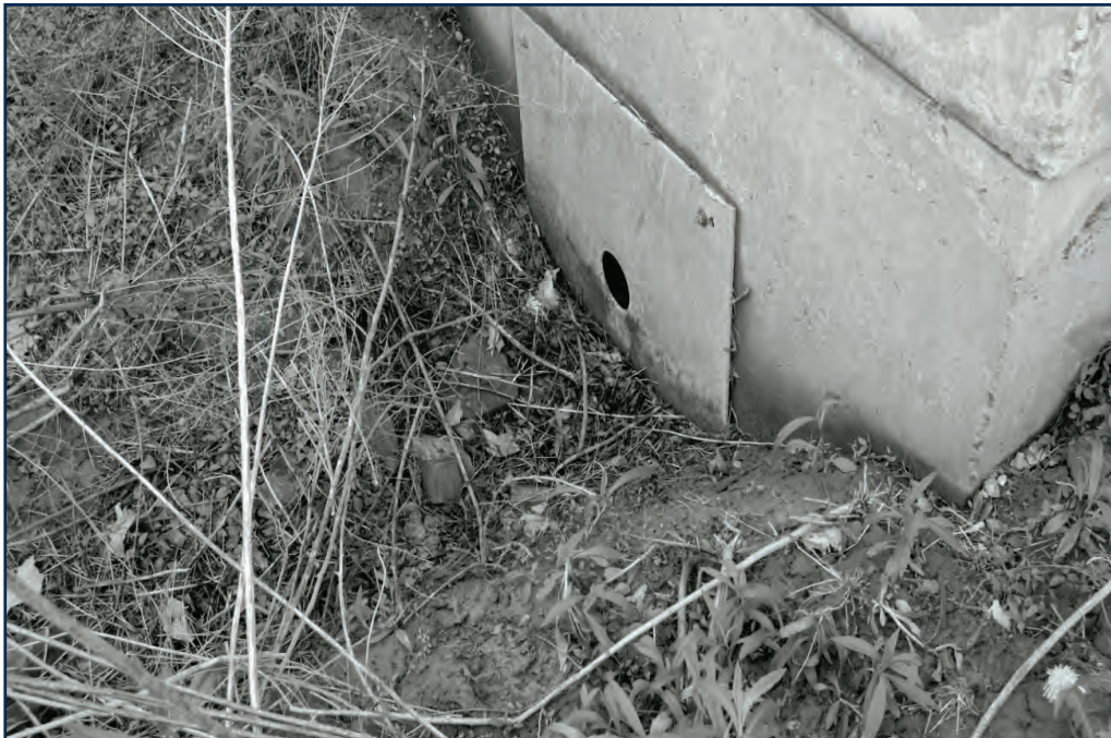
Figure 14: Conventional stormwater basin located along Township Line Road (May 2013)
