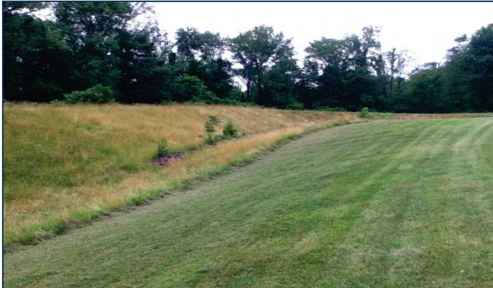
Figure 2: Elongated detention basin at the Shrine of Czestochowa (July 2013)
