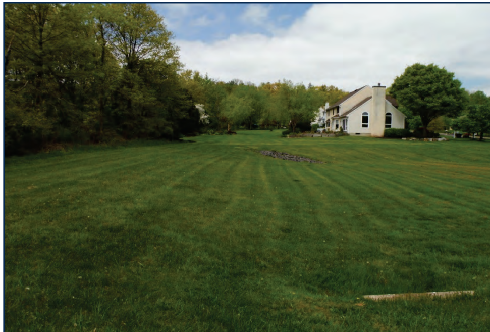
Figure 7: Detention basin at Hagan Court Subdivision (May 2013)
