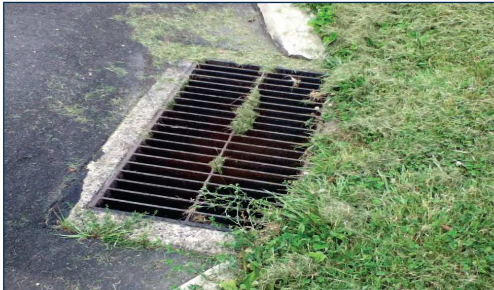
Figure 3: Stormwater catch basin that could be retrofitted with a Manufactured Treatment Device at the Shrine of Czestochowa (July 2013)
