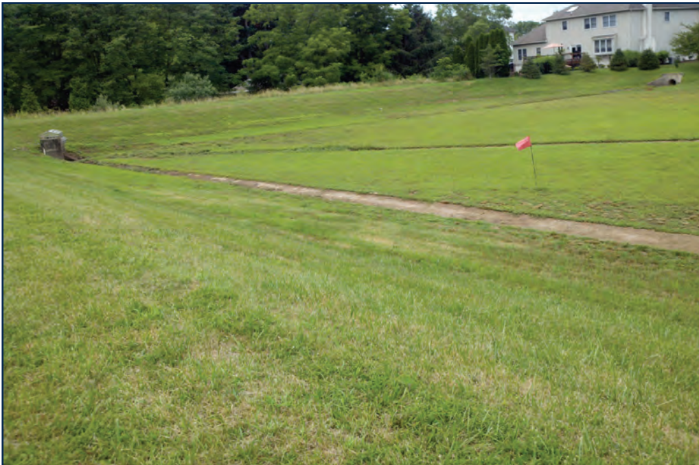
Figure 12: Low flow concrete channel at bottom of basin along Redfield Road (July 2013)
