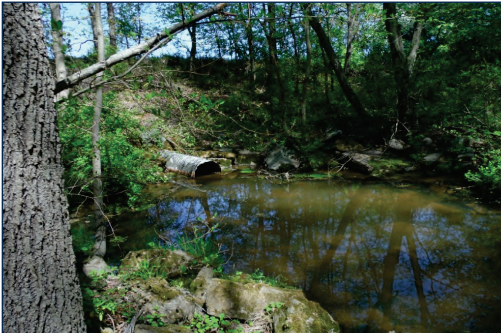
Figure 5: Below Pine Run Reservoir (May 2013)
