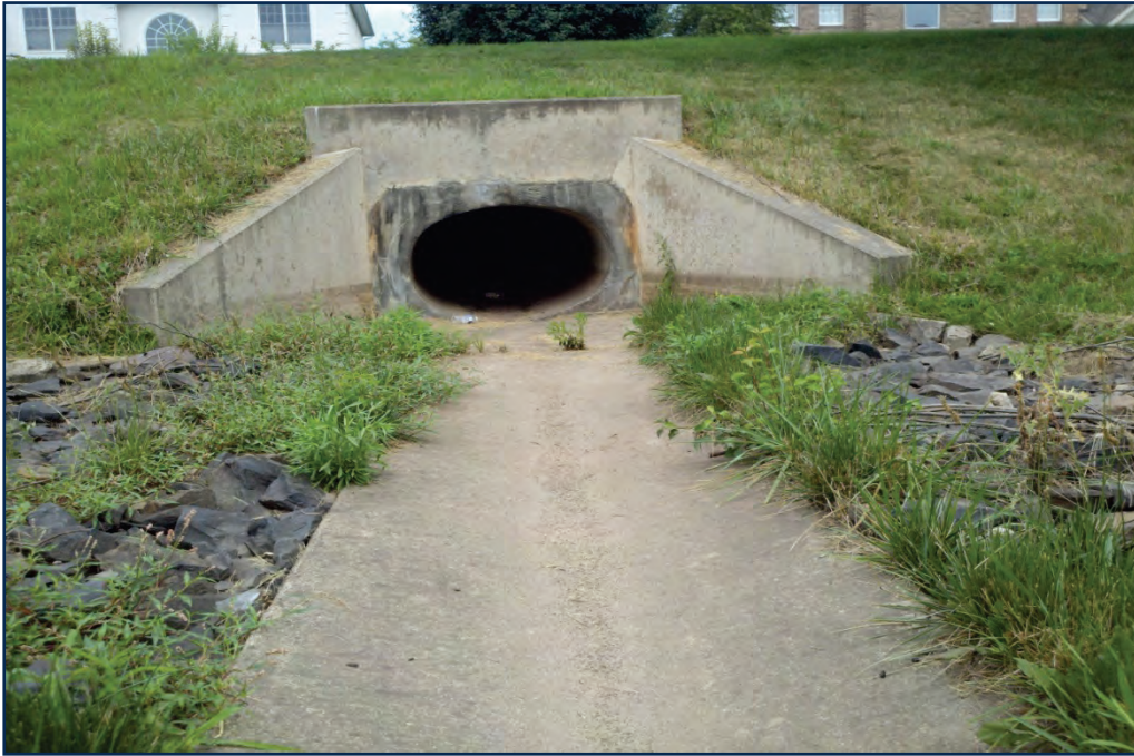
Figure 11: Large outlet pipe for a basin along Redfield Road (July 2013)
