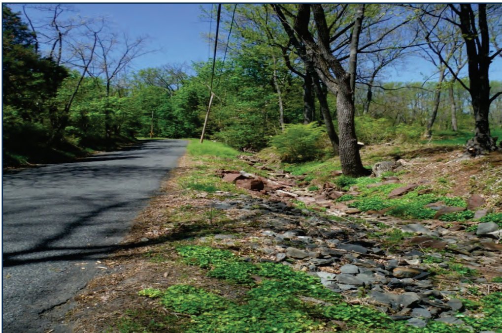
Figure 8: Roadside swale along Pine Run Road (May 2013)
