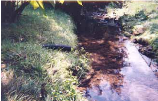
Photo 3. Drain pipe for stormwater discharge.
