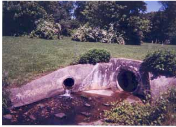
Photo 4. Pond outlet & detention basin outfall
