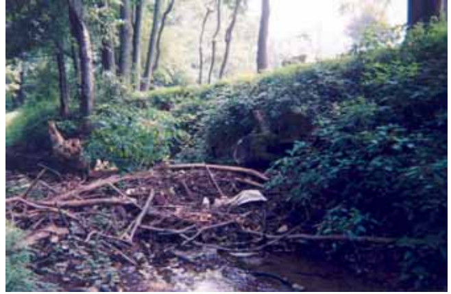
Photo 2. Severe erosion and debris dam.
