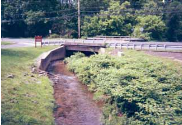
Photo 1. S. Branch flowing under Bristol Rd.
