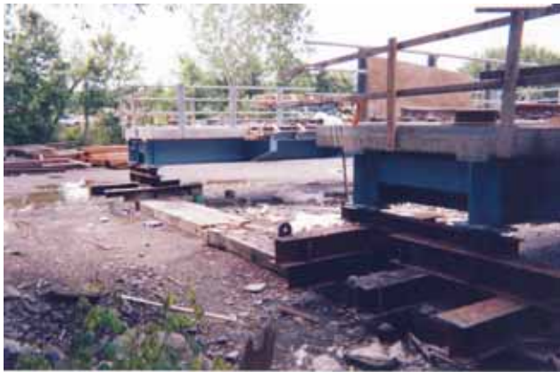
Photo 9. Poorly maintained industrial lot
