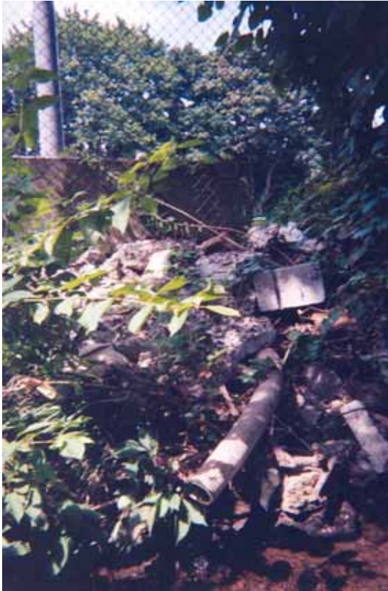
Photo 1. Commercial parking lot stormwater discharge pipe.
