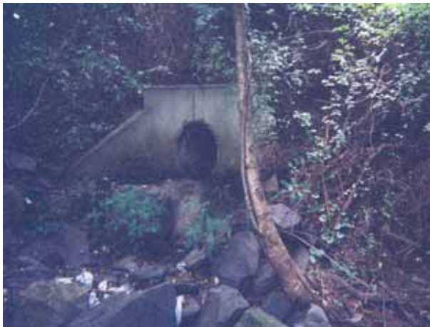
Photo 5. Storm sewer outfall.
