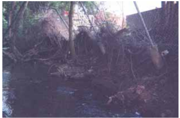
Photo 10. Erosion undermining fencing
