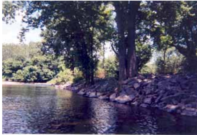
Photo 4. Boulders stabilizing streambanks
