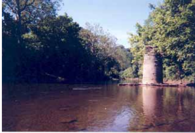
Photo 2. Abandoned bridge abutment
