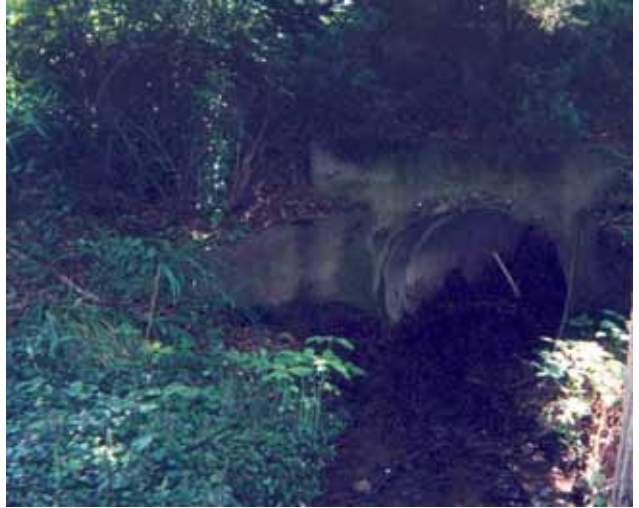
Photo 2. Storm sewer outfall
