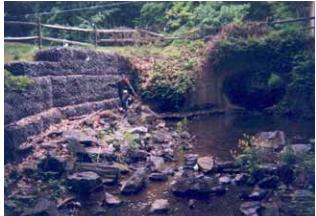
Photo 4. Bridge over Old Jordan Road
