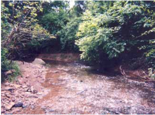
Photo 7. Exposed stream banks
