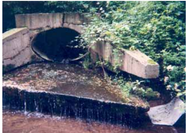
Photo 4. Storm sewer discharge
