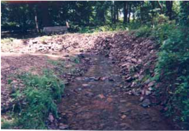
Photo 3. Attempt at erosion control
