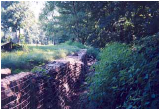
Photo 3. Gabions stabilizing streambank
