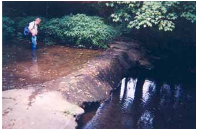
Photo 4. Dam across Pine Run
