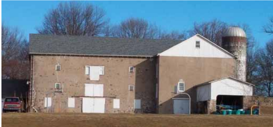
Worth Barn at George School
