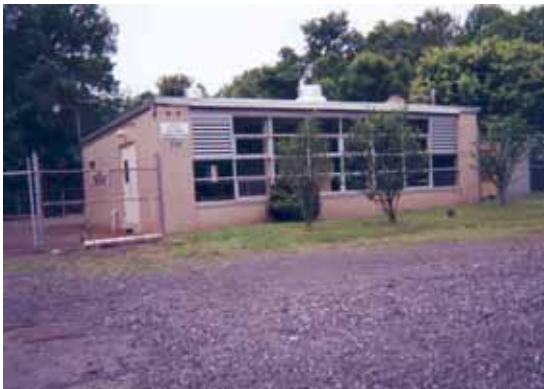
Photo 11. Mill Creek pump Station
