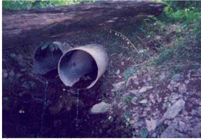
Photo 1. Dry weather discharge from storm water pipe
