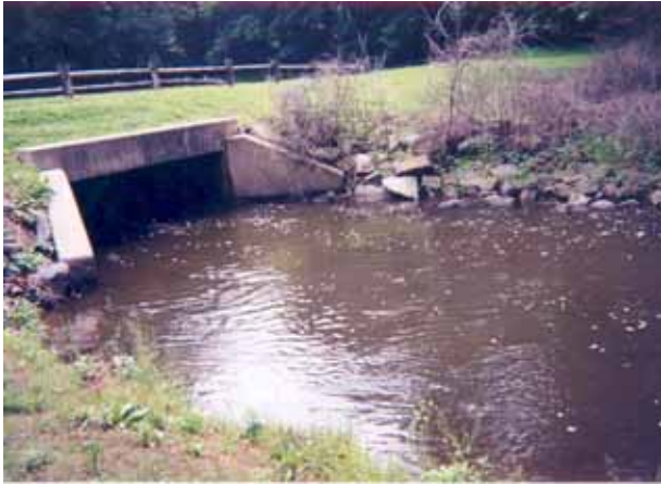
Photo 1. Core Creek under Park Road
