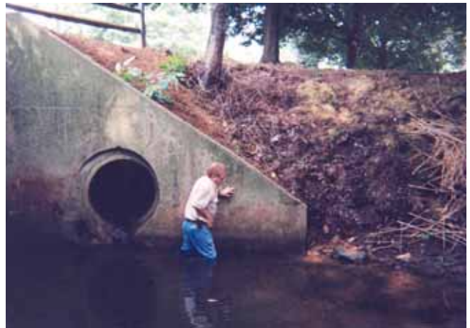
Photo 6. Storm sewer outfall at Woodenbridge Rd.
