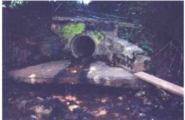
Photo 4. Discharging storm sewer
