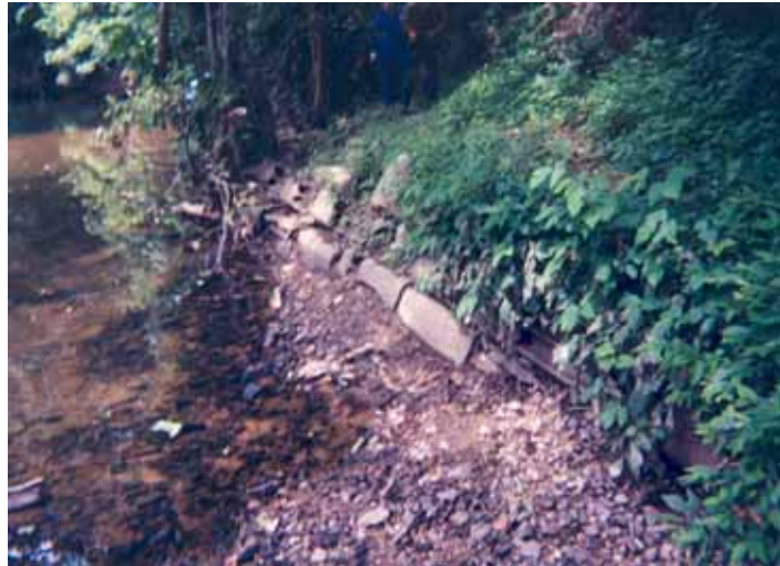
2. Concrete pipes stabilizing streambank
