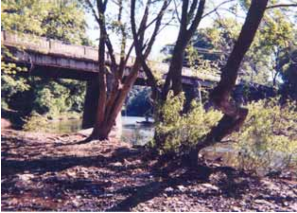
Photo 1. Newtown-Richboro Road Bridge
