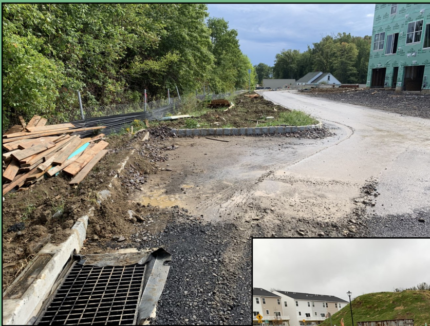
It's difficult to distinguish because of how damaged it is, but the crushed, black "tube" at the very bottom of the photo at right used to be a functional compost filter sock. These are installed to keep sediment on site and prevent it from washing into local waterways. However, they don't work well when they're destroyed by construction traffic. BCCD made sure these controls were reestablished.
