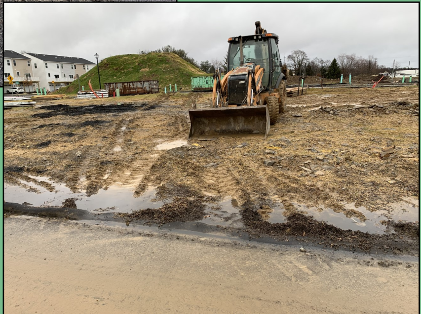
It's difficult to distinguish because of how damaged it is, but the crushed, black "tube" at the very bottom of the photo at right used to be a functional compost filter sock. These are installed to keep sediment on site and prevent it from washing into local waterways. However, they don't work well when they're destroyed by construction traffic. BCCD made sure these controls were reestablished.
