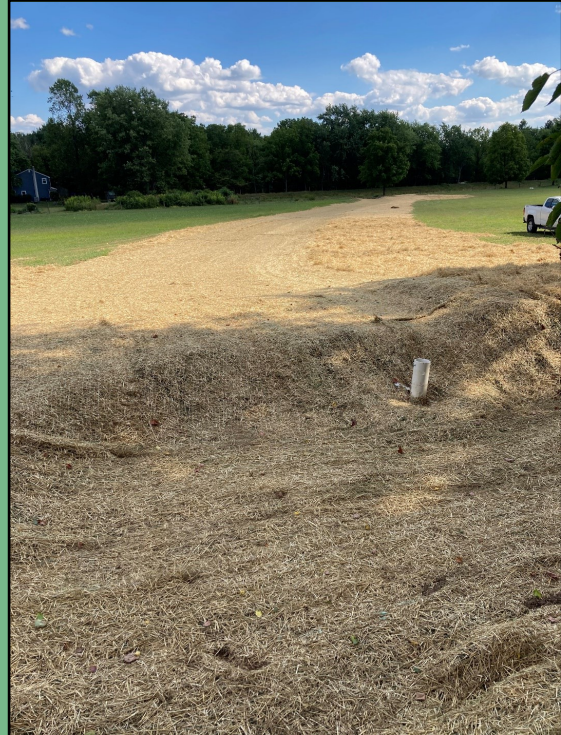
Above: Photo of a stormwater and sediment control basin outletting into a grass waterway. This was installed to address gully erosion in the crop field caused by upslope stormwater from a housing development.
