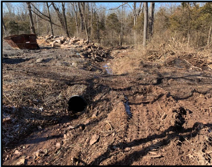
The photo at right shows a discharge pipe into a sediment control basin. Though basins are designed to handle sediment discharge from standard rainfalls, the sediment delta deposition at the discharge of this pipe indicates that there are site issues “upstream.” BCCD worked with the site developer to address conditions so that excessive amounts of sediment were not discharged into the basin and ultimately off site.
