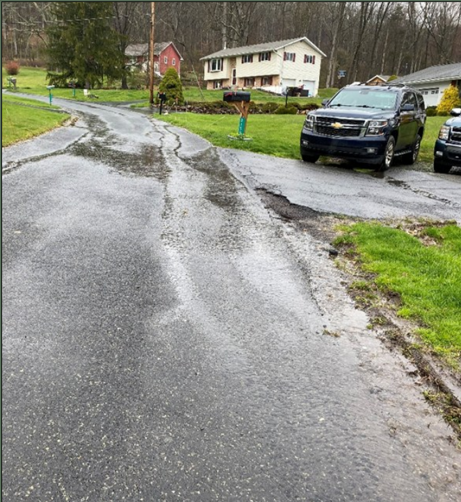
Photographed above is an area on Lakeview Drive that houses were at risk from flooding due to road surface and drainage issues.
