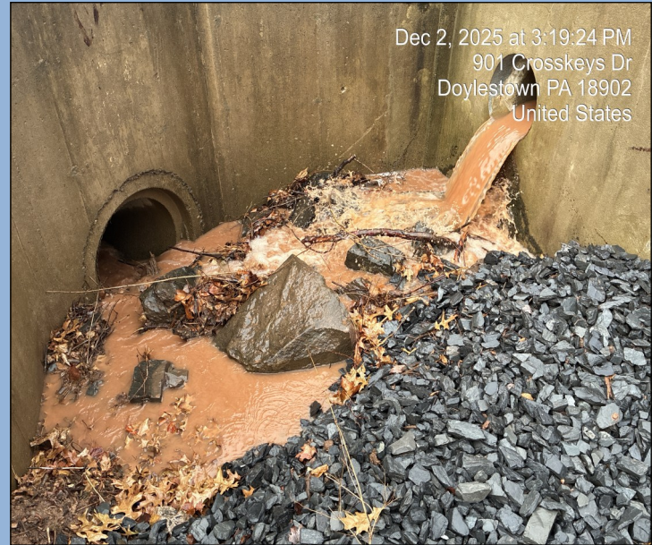
Observed above is sediment-laden discharge into a local stream from complications on one project site.
